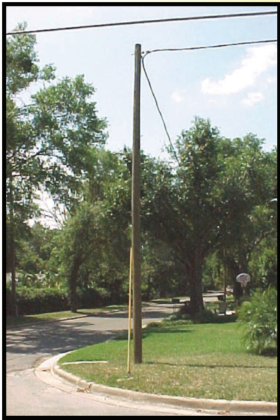
Temporary New Poles Installed
